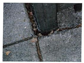
ITEM 6 Fungus has damaged the lower base framing at the area indicated on the diagram.
